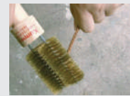
3. Clean the surface of conductor and rod by cable clean brush and preheat by butane torch to ensure the conductor is totally dry
