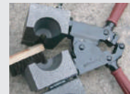
9. Gently rub slag from the crucible by scraper. Clean the crucible and weld cavity by mould cleaning brush to endure the mould
