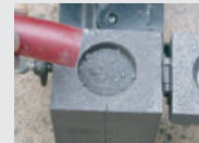
6. Pour a recommended size of weld metal into the mould crucible. Check for leaks of weld metal. Repeat step 4 in case of leak
