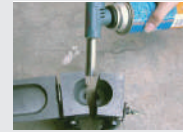
2. Preheat by butane torch to ensure the mould is totally dry
